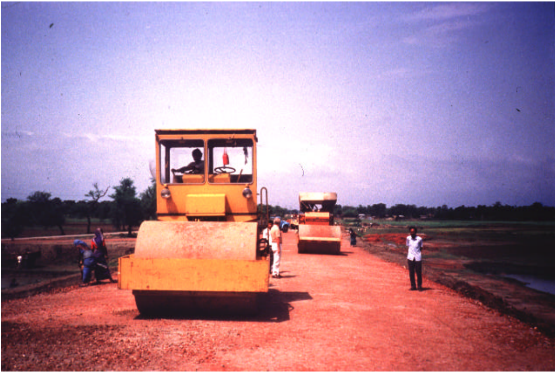
Photo 1. Rolling Pavement Layers, suitable and adequate compaction equipment must be used.
