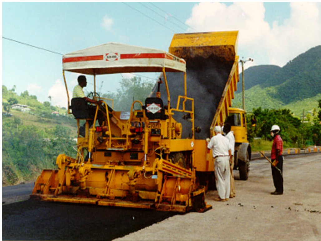
Photo 6. Truck Containing Asphalt backing up to Paver.
