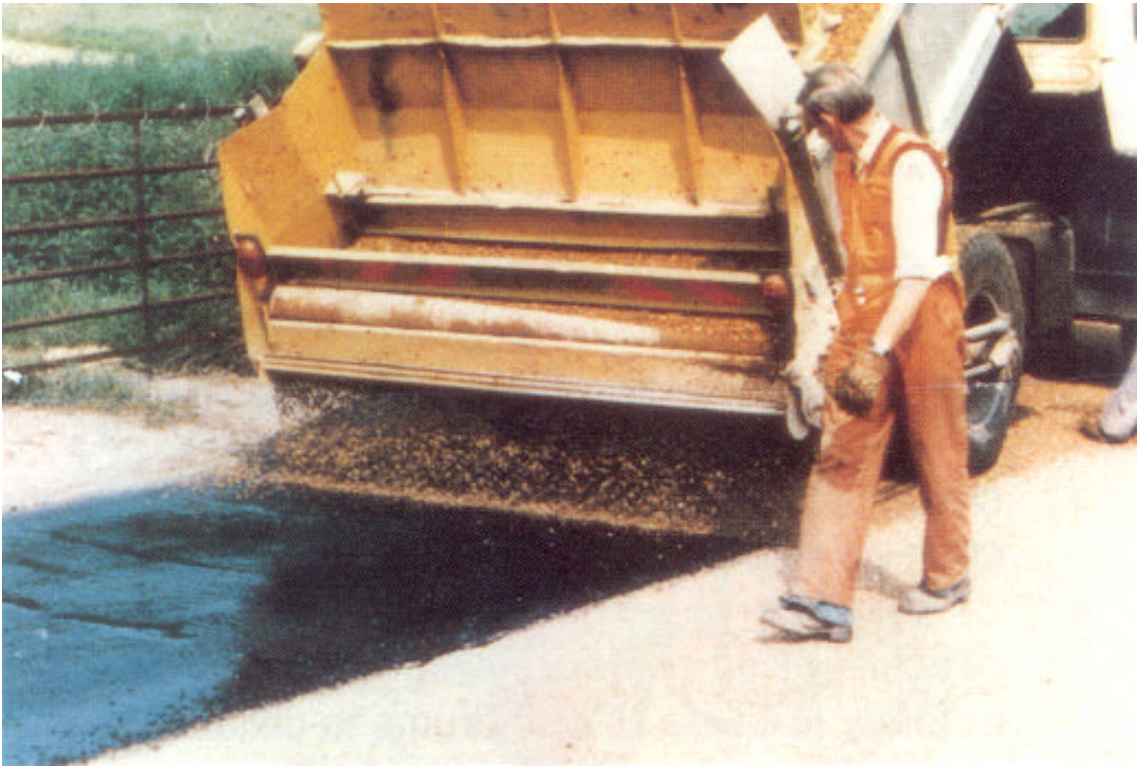
Photo 3. Mechanical spreader spreading aggregate on recently sprayed bitumen surface.
